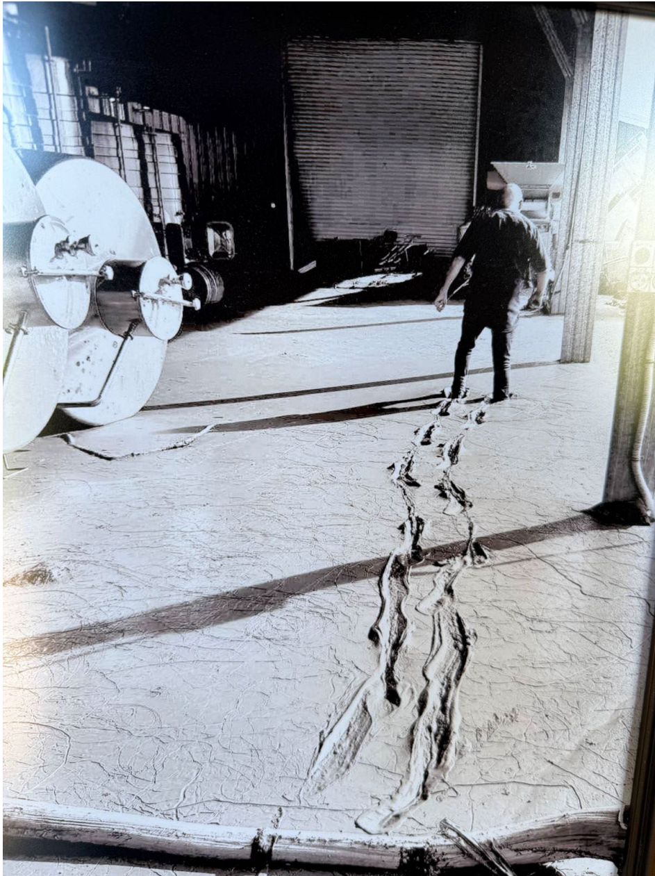
Figure 6 Kel Dixon, Winemaker, Shed 530, Winery immediately post Cyclone.
